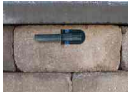
Figure 6.5 – Fasten down the bracket
