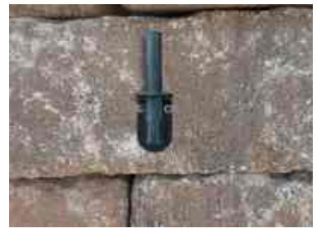
Figure 6.8 – Dry fit the bracket
