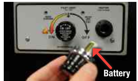
Figure 10.6 – Slide battery into spark igniter unit.
