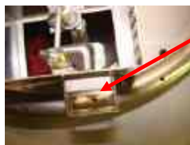
Pilot Window lined up with burner hole.
