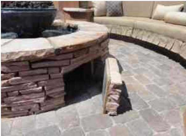
Stone enclosure on site
